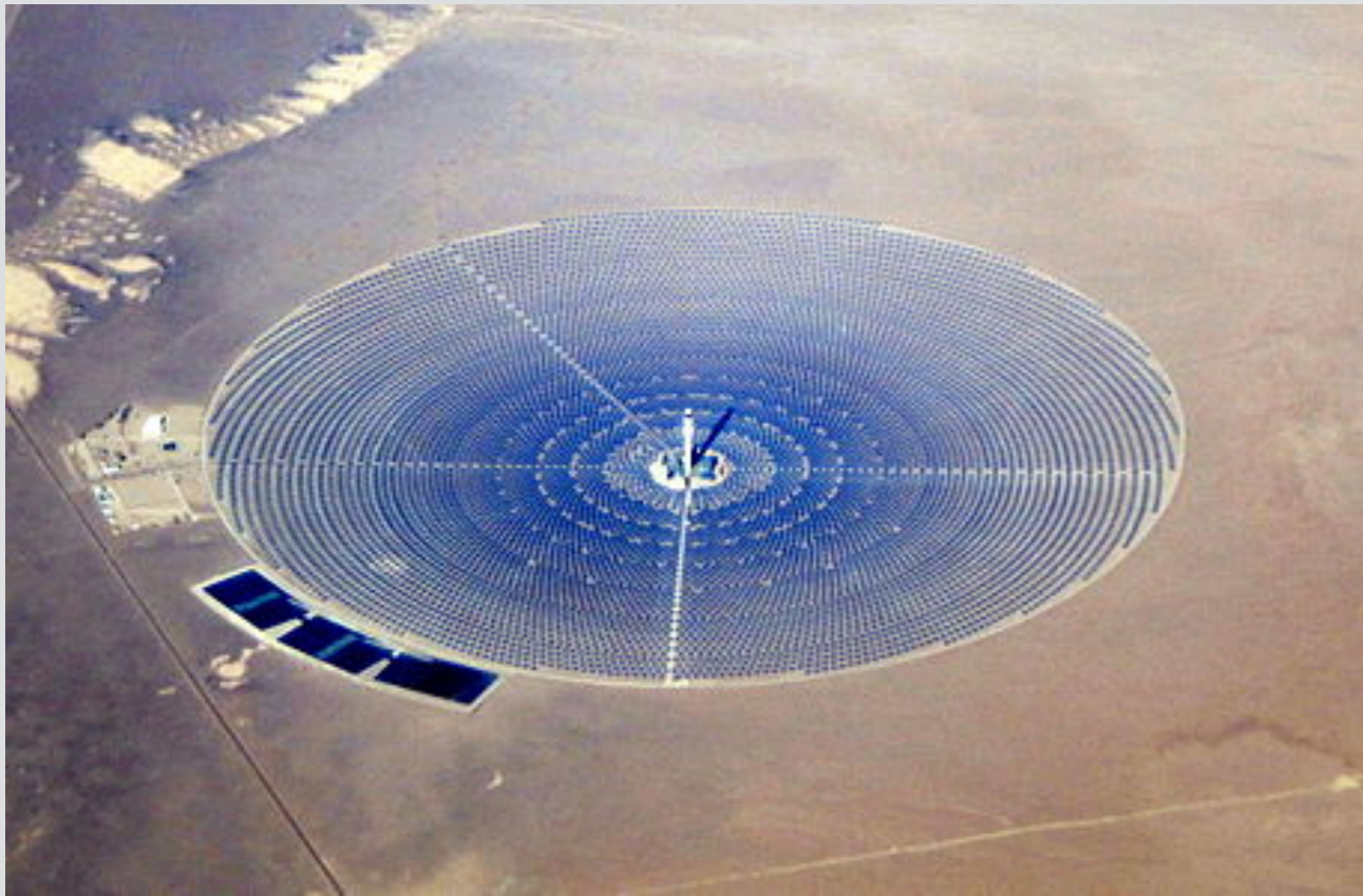
Crescent Dunes solar collector 1.25 km diameter
